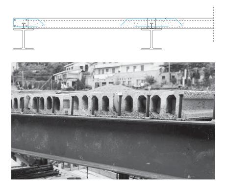
Fig. 4.22 Hollow core floors on steel beams. Connecting rivets can be induction-welded to the upper flange of the beam even after the laying of the slabs.
