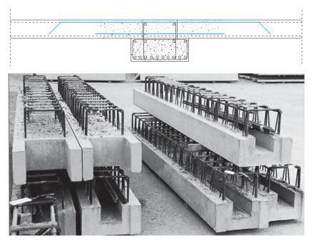
Fig. 4.21 Semi-precast beams of normal or prestressed concrete. The beam-floor connection must always be a continuous, or at least partially continuous, restraint.
