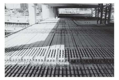
*Fig. 4.16* Slab end prepared for casting of a fairly large corroborant flange
