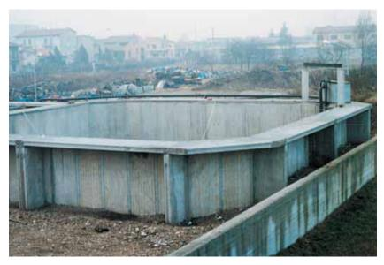
Fig.1.3 The hollow core walls of a water treatment tank
